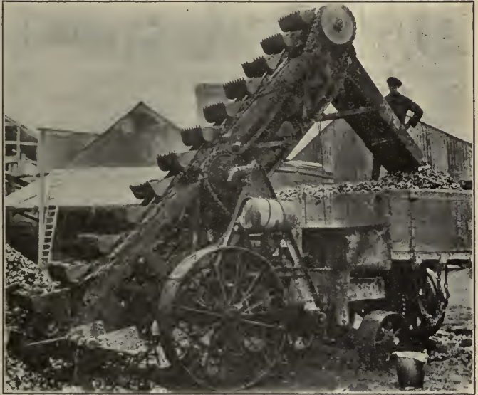
LOADING TAR MACADAM BY MACHINE
